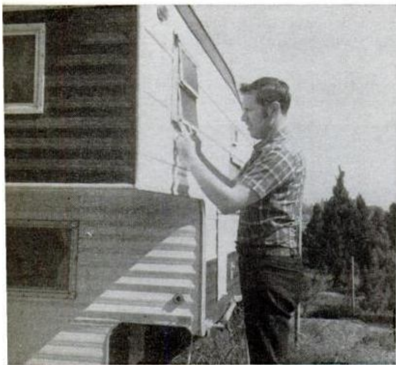
CHECK ALL WINDOWS AND DOORS. This frame had been bent and the window would not close all the way. Result: cold drafts down my neck. Straighten faulty hinges and moldings; if necessary, replace them
